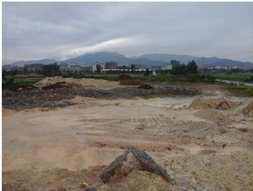
Source: Fujian Fuqing Project
