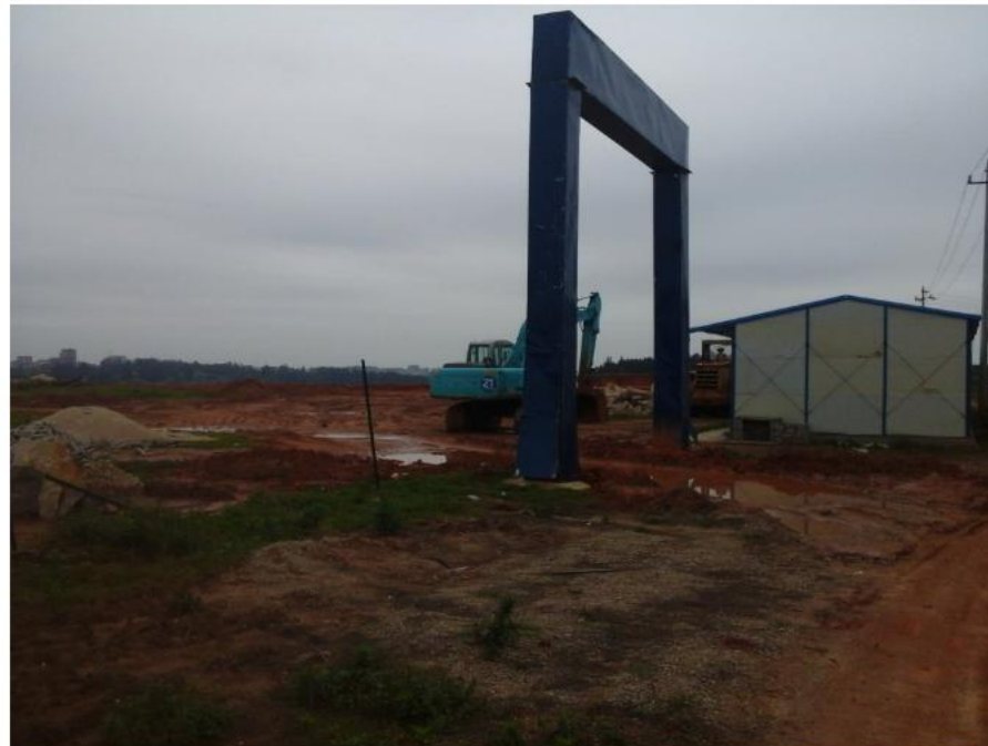
Source: Fujian Fuqing Project
